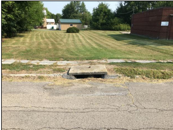
Typical Existing Street Catch Basin
