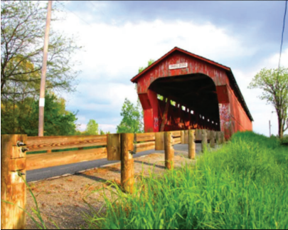
Swartz Bridge, Wyandot County, Ohio
