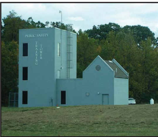
New Public Safety Training Tower on Reed Street
